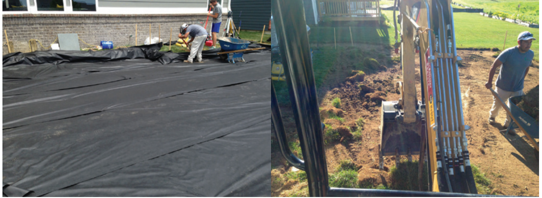
In progress shots detailing the progress of the project.
